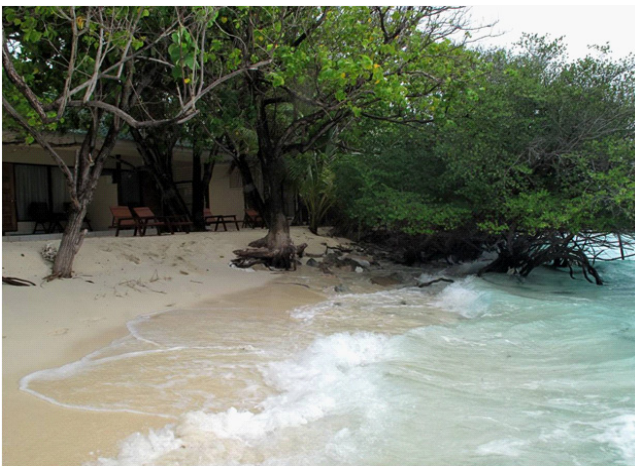
Figure 5 During high tide with strong westerly wind the sea washes with several meters of the villas, North Male' atoll, October 2009
